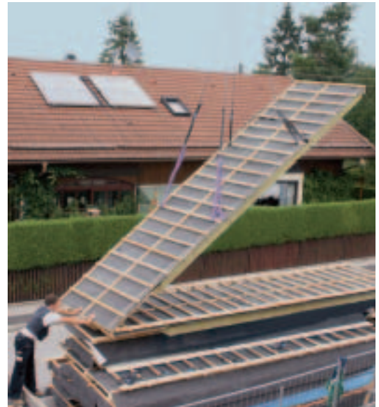
Montage Finnroof-Elemente
